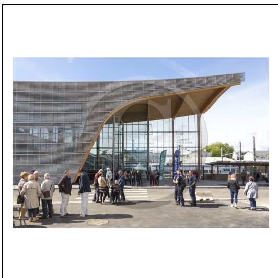
Inauguration de la gare de Lorient le 20 Mai 2017***Inauguration of the Lorient train station on May 20, 2017
